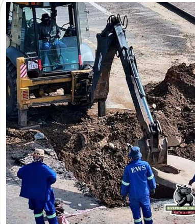
eTM service delivery work
